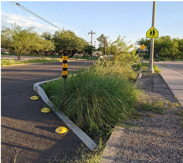
Figure 3. This streetside chicane planted with native shrubs, trees, and grasses collects runoff during rain events. Grass species are emphasized as their roots are quick to establish, and they help to break up the soil, encouraging infiltration. Grasses also aid in the filtering of runoff. Grass species included in this planting are Bouteloa gracilis , Bouteloa curtipendula , and Muhlenbergia emersleyi . (Design: Tucson Clean and Beautiful. Construction: Desert Living. Maintenance: Neighbors)
